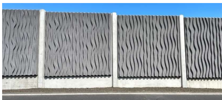
Fig. 6.11 Concrete noise reduction barrier
