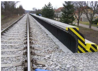
Fig. 6.1 Low noise barrier [19]
