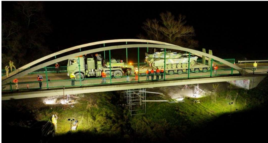
Fig. 8 Full military load on the bridge (105 t) Source: Photographed by Dominik Mák.
