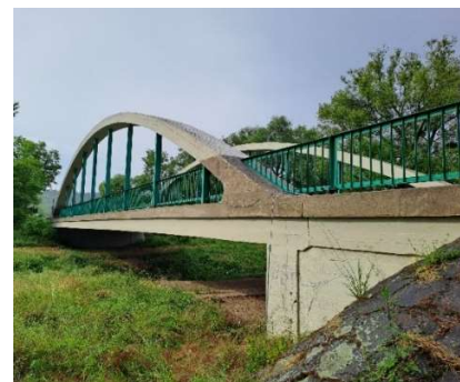
Fig. 1 View of the selected bridge Source: Photographed by Benedek Kapin.
