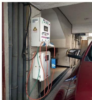
*Figure 12 Personal charging point in a housing society*
