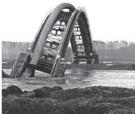
**Figure 4.** Destruction of the supporting structure of the bridge during the floods in 1974 on the Slaná River.
