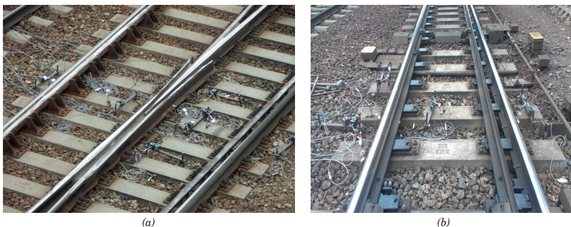
Figure 2 The view of the common crossing (a) and a switch (b) unit of turnout
