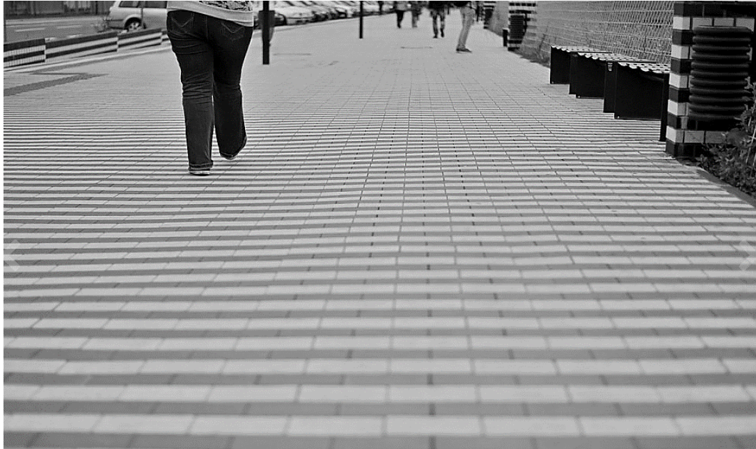
Fig. 2 Unsuitable use of material combinations (Source [1])
