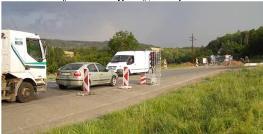
*Fig. 4 The use of a mobile lighting signalling device and traffic signs (archive of authors)*
