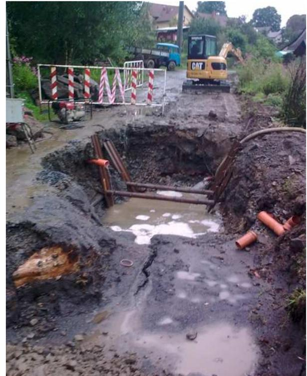
*Fig. 1 Incorrect fall-prevention measures at an excavation (archive of authors).*
