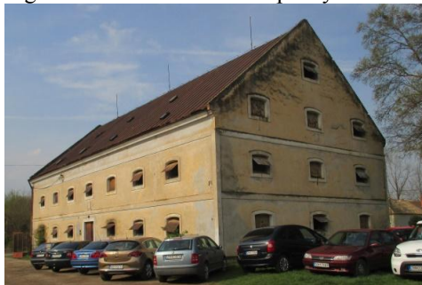
Figure 14: Brownfield in Slepčany
