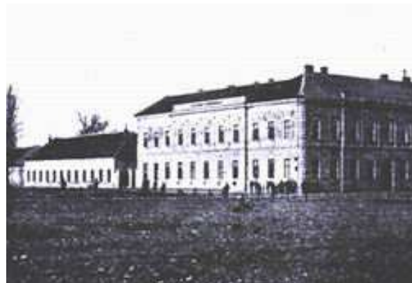
Fig. 5 Building of the Higher Mechanical Industry School in Košice.
