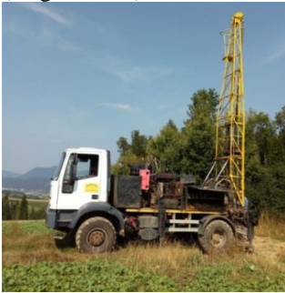
Figure 3: Core-drill rig at Site 2 (August 2018)
