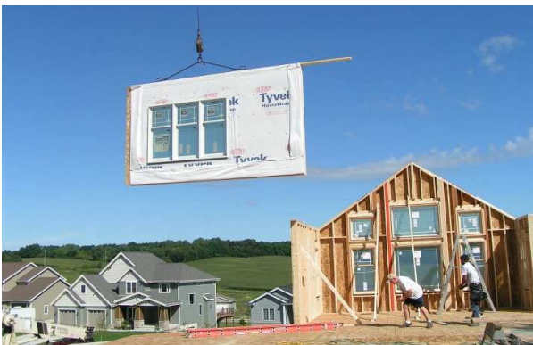
Fig. 2 Panellised construction [9]
