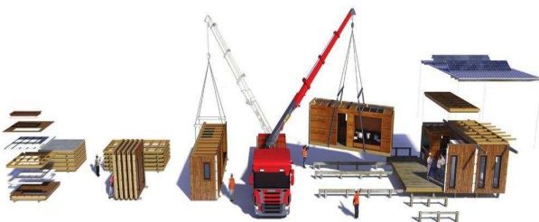
Fig. 3 Hybrid construction [10]
