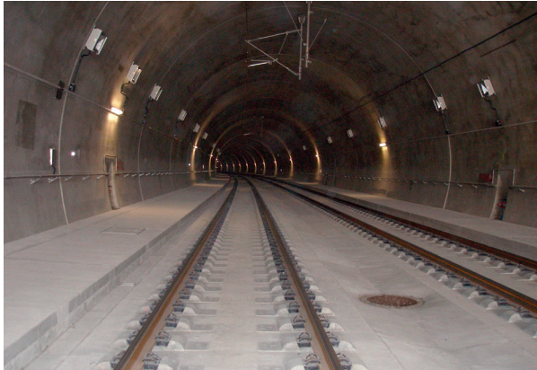
Fig. 1 Type of Ballastless Track Construction RHEDA 2000
