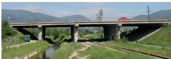
Fig. 1 The view of bridge No. 018-293 near the town of Martin on I/18 road
