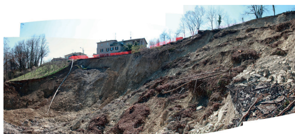
Fig. 3 Boschetto landslide’s crown area. The provincial road that crossed the slope just in front of the depicted house was completely destroyed by the landslide, causing the seclusion of the inhabited upper Parma river valley
