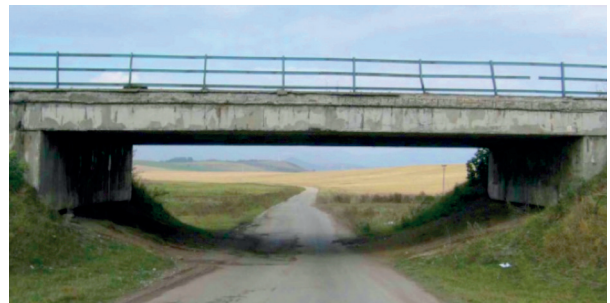
Fig. 3 The view of bridge No. 065-086 near the village Mosovce
