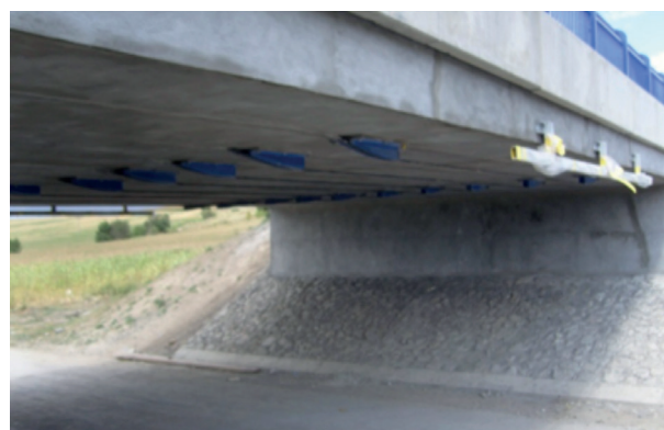
Fig. 10 Bridge No. 065-086 after strengthening by external prestressing
