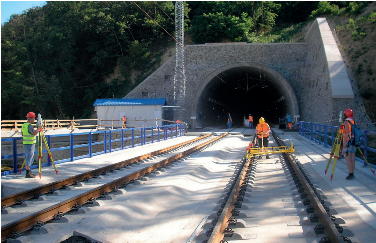
Fig. 5 View of the slab track structure of the railway bridge (diagnostics of actual and relative position of the track realized)
