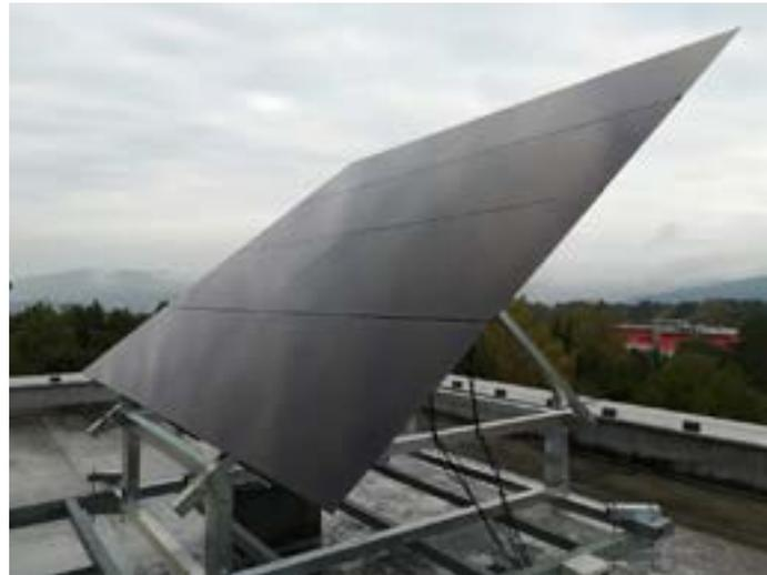
**Figure 5** The PV string installation on the University Science Park's roof in Zilina, Slovakia
