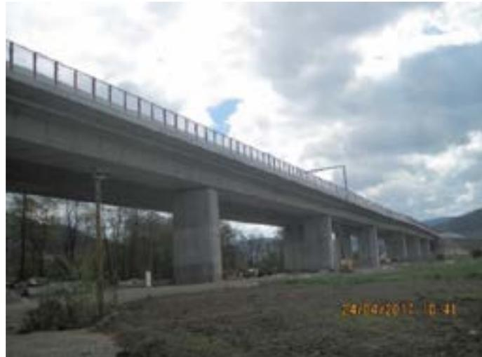
**Figure 1** Overall view of the tested ten-span continuous concrete box-girder bridge
